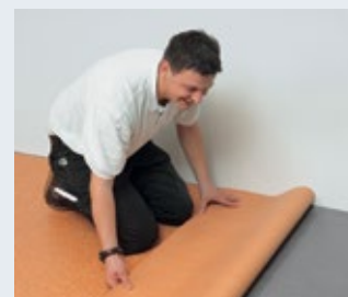
4. Lay in new flooring and press down avoiding stress or distortion
