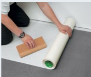
2. Bond Sigan 1 on the prepared subfloor
