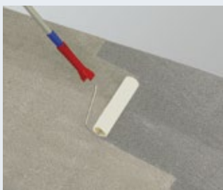
1. Apply special Primer Planus on the subfloor
