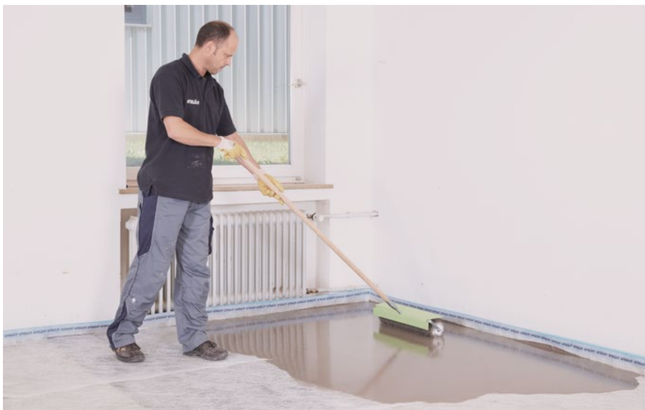
Installation of the Self Levelling Cementitious Thin Screed UZIN SC 927
